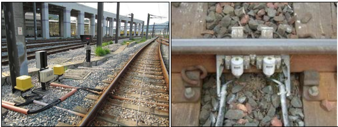
Figure 20: Axle Counter Installation (Left) and Detector Head (Right) (Sin, 2013a)
